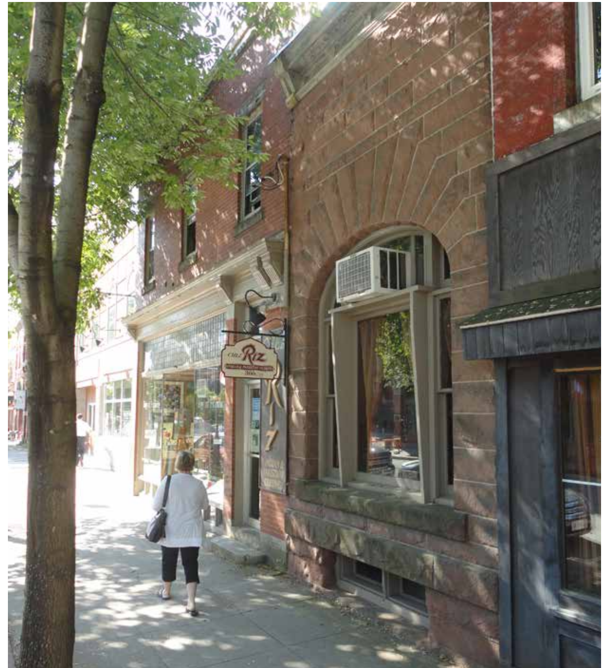
Heritage fabric of Queen Street
