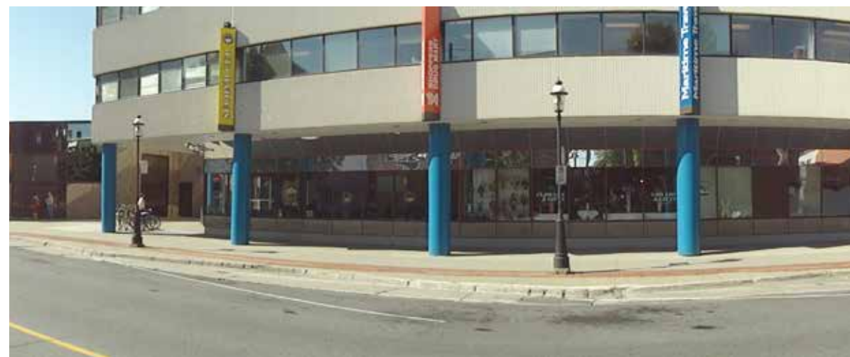
Existing condition of the Kings Place Shopping Centre fronting on King Street
