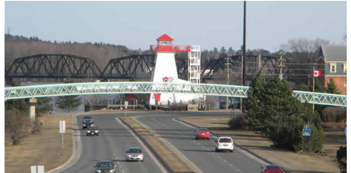
St. Anne's Point Drive in its current condition
