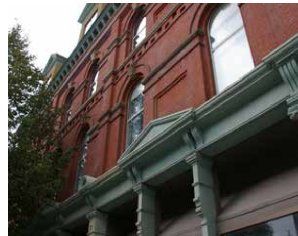
Architectural character of Queen Street
