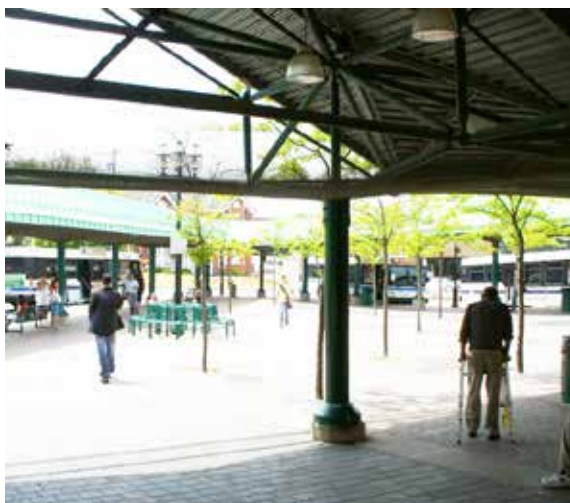
Integrated transit facility in Barrie, Ontario
