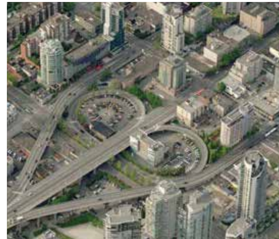
Existing Granville Street Bridge
